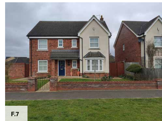
Figure 07: Footpath tucked behind a grass verge to add a greater element of safety.
